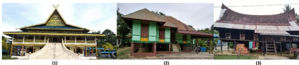
Figure 5. The types of roof shapes on the Riau Malay vernacular house: (1) Gable/folding awning roof, (2) Pyramid, (3) Lontik
