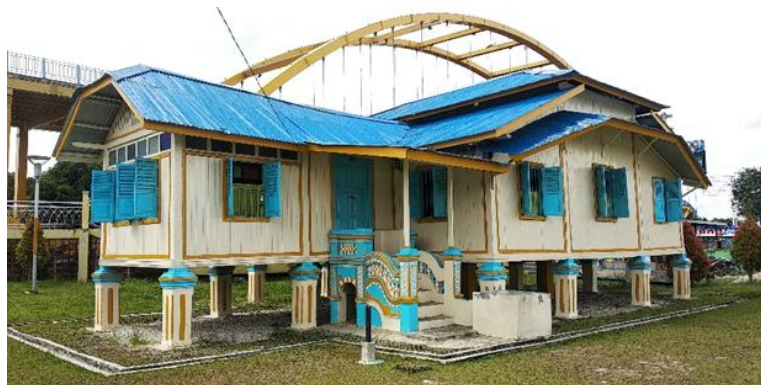
Figure 2. House of the Judge ( Rumah Tuan Kadi ) on the Siak riverbank at Kampung Bandar, Pekanbaru City
